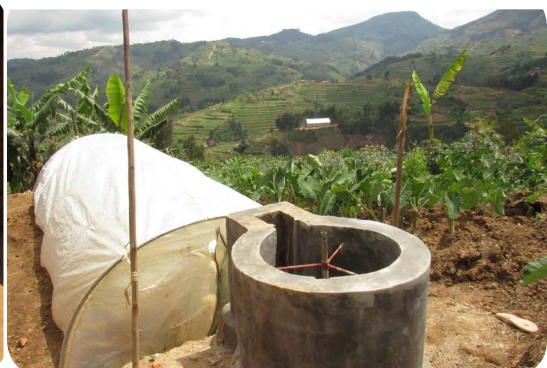
A Canvas-type biogas digester under construction in Rutsiro District, Rwanda
